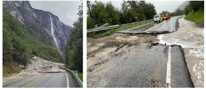
There has been a large number of damaged roads after "Hans" – both mudslides caused by the extreme weather and flooding. Photo: Norwegian Public Road Administration/Asbjørn Stensrud
